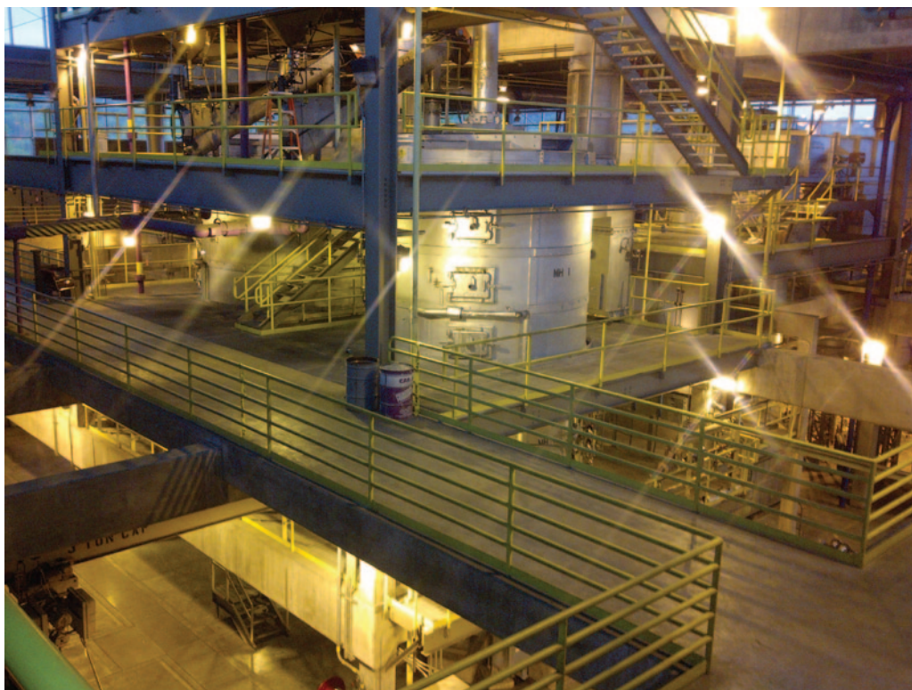
Multiple Hearth Furnace
